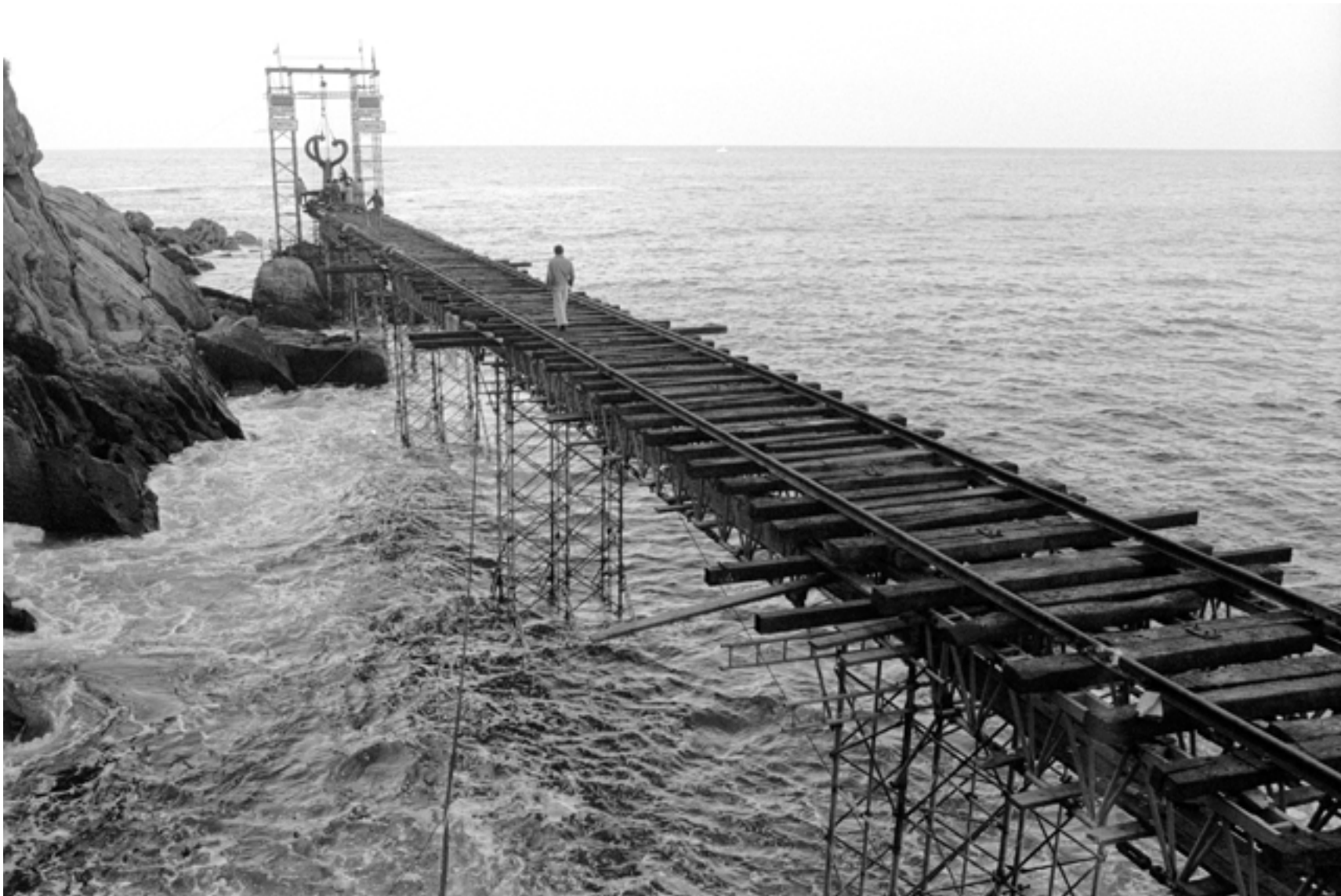
Installation of one of sculptures. © Jesús Uriarte
